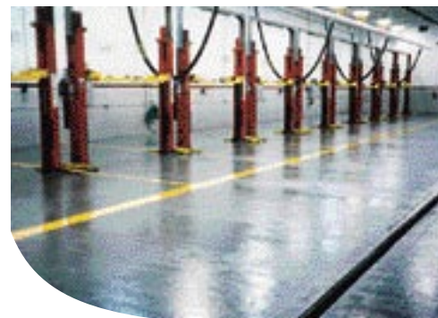
AUTO SERVICE BAYS/FIRE STATIONS Decorative Quartz Floor
