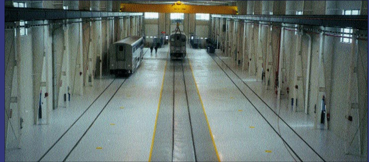
C.A. REED ASSOCIATES, INC. • INDUSTRIAL FLOORING SPECIALISTS
