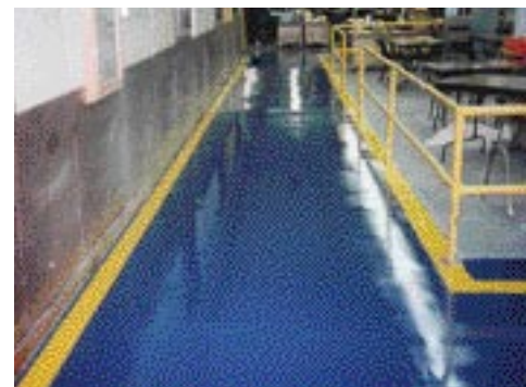
AISLE RESURFACING Industrial Epoxy Topping
